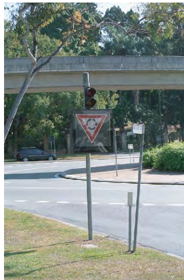
(c) Combination metering signal and changeable yield sign Brisbane, Queensland, Australia
