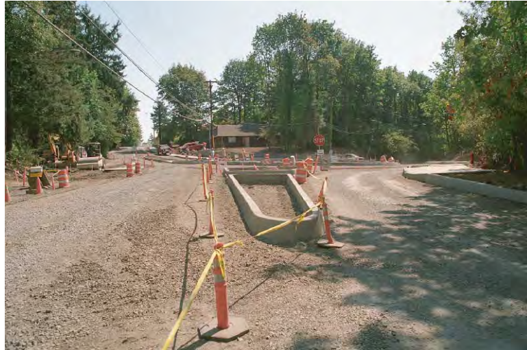
(a) Splitter island construction (Portland, Oregon)
