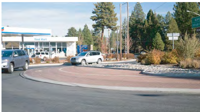
(b) Maintenance pullout in central island (Bend, Oregon)
