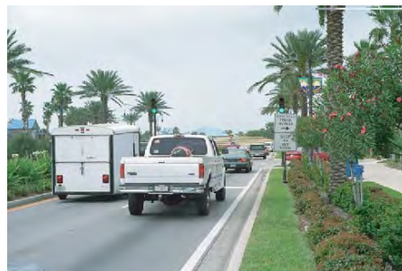
(a) Approach metering signal Clearwater, Florida
