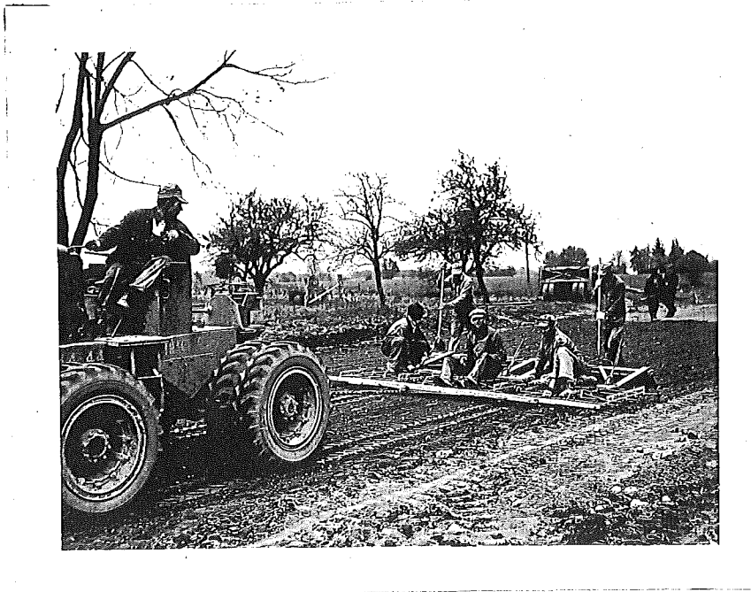
a. Dragging to remove surface compaction planes and produce a mulch.
