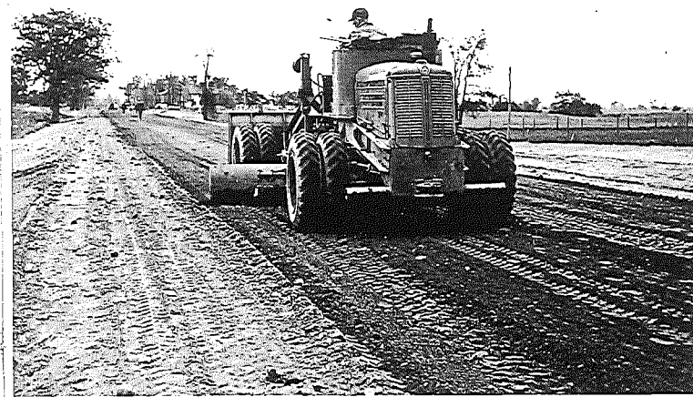
d. Final shaping with the patrol grader.
