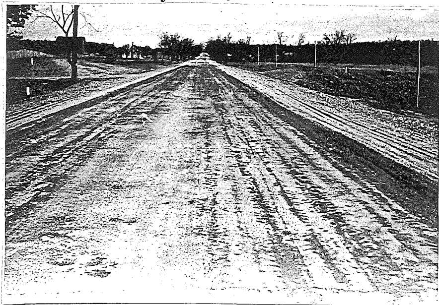
c. General surface condition Station 95+00 Surface in good condition.
