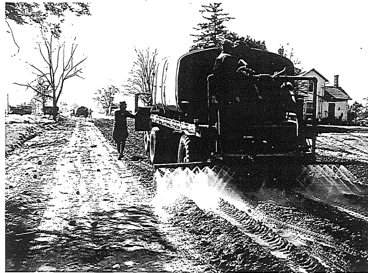
b. Adding water with the distributor.
