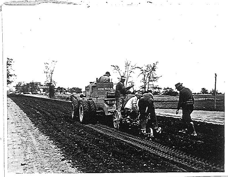
d. Mixing with the three-gang plow.
