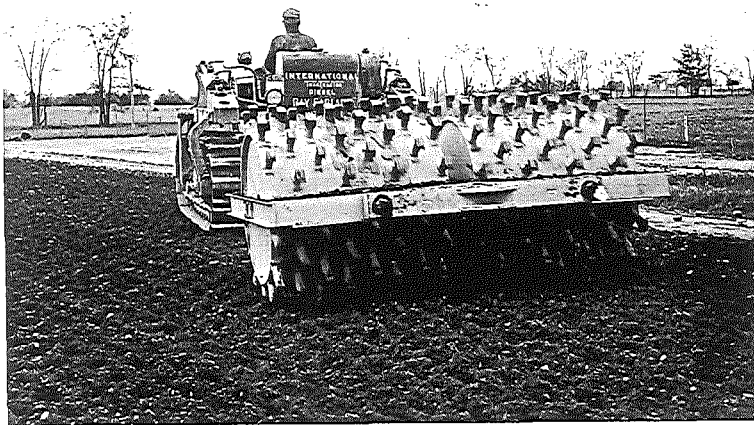
c. Compacting with the sheepfoot roller.
