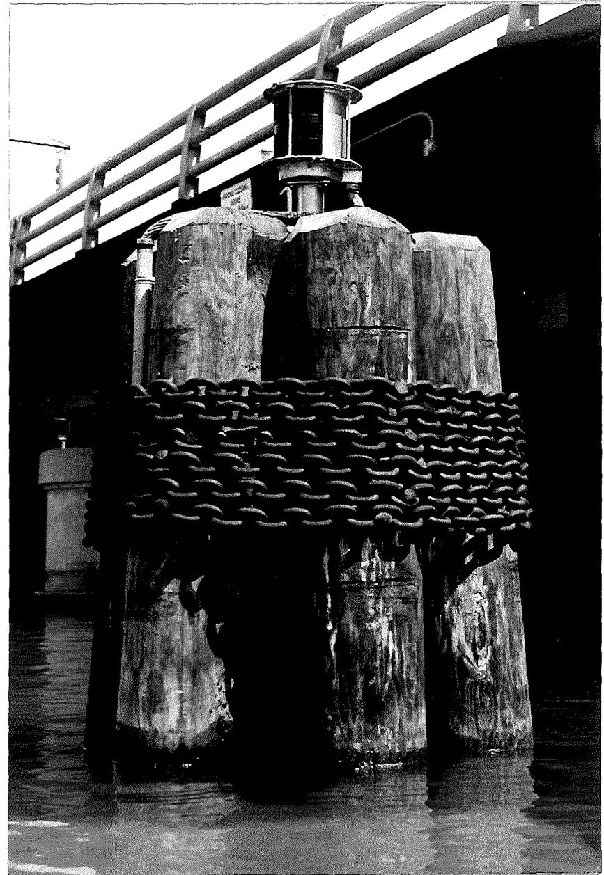
Figure 4. Pile cluster 3, treated with Osmosalts, viewed facing northwest (left) and northeast (right).
