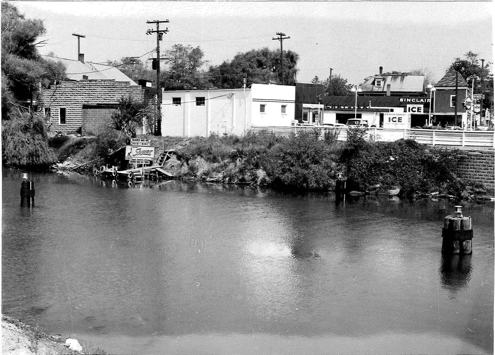
Figure 1. Three of six new pile clusters near M 29 bridge over Pine River, St. Clair. View facing northwest showing piles treated with creosote (Nos. 1 and 2) and Osmosalts (No. 3).
