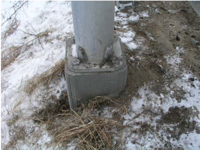
Figure 6. Dig out and regrade slope.
