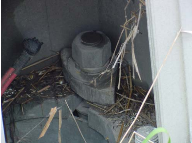
Figure 2. Steel screw-in foundation in the vicinity along US-131
