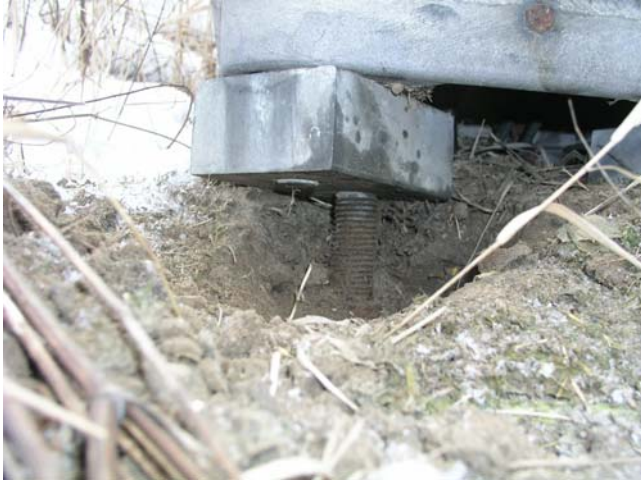
Figure 12. Place on new foundation.
