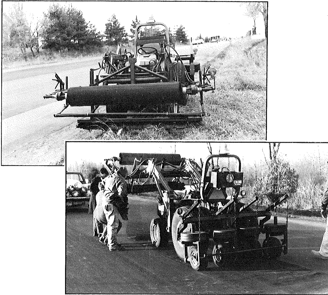
Figure 2. Modified tractor for installing the Glasgrid.
