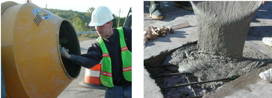
Figure 3.6 Demonstrations of ECC workability in patching of a bridge deck for (a) mixing in a 12ft<sup>3</sup> capacity drum mixer; and (b) pouring without any vibration.
