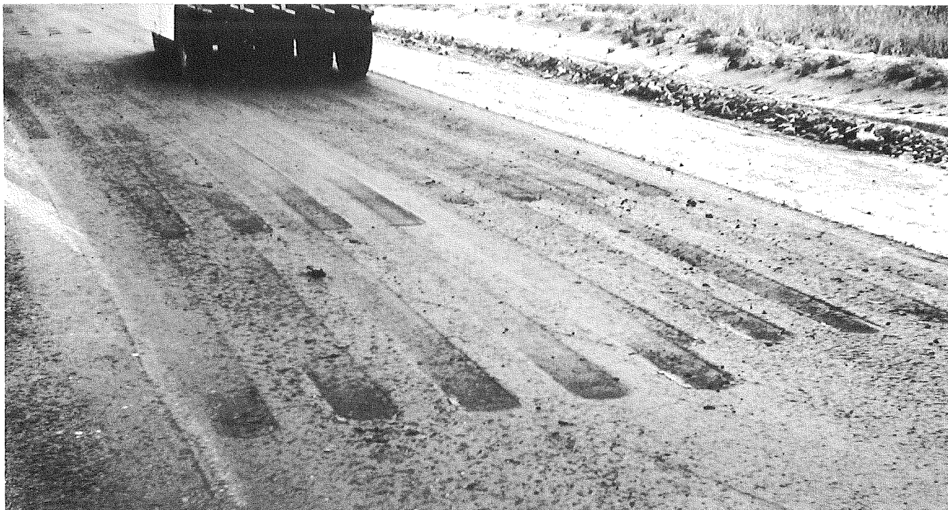
Figure 12. Showing chatter or scuff marks produced when pneumatic tire roller starts too quickly.
