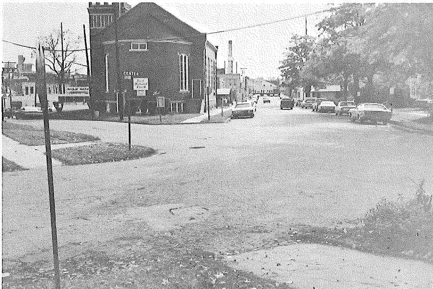
SOUTHBOUND COMMERCIAL STREET
