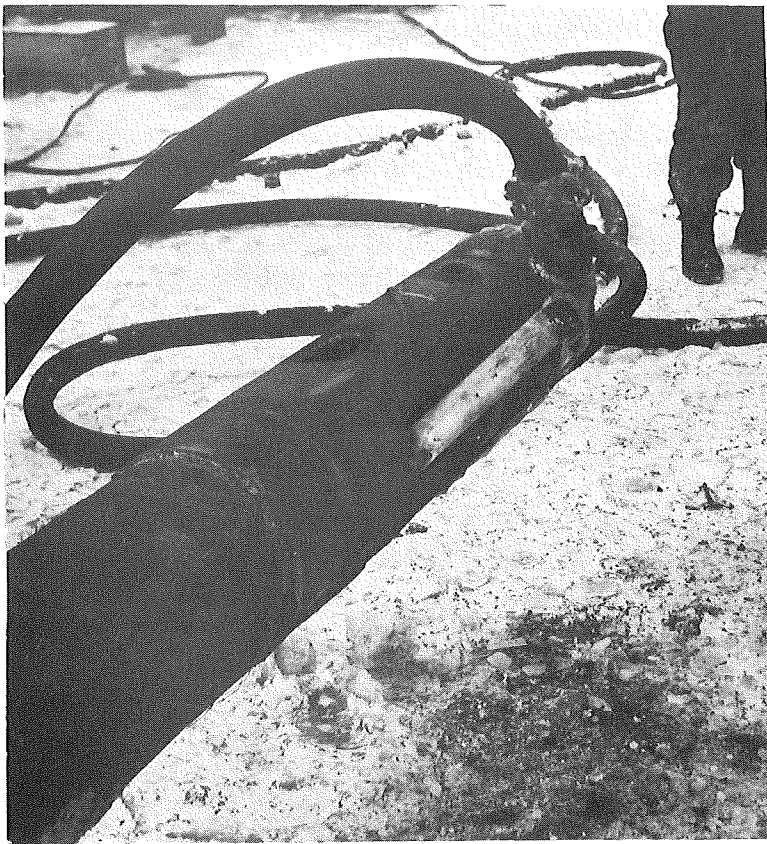
Figure 97. Internal jetting of open-end pipe piles during driving originally involved a system having a jet pipe fixed in the follower (upper left) with an inlet connection elbow fixed by welding; this follower assembly was then welded to the pile (upper right). The second system fabricated (lower left) had a floating, non-fixed jet pipe, allowed to protrude through an open port in the follower side; spoil flowed through ports when the assembly was in operation (lower right).
