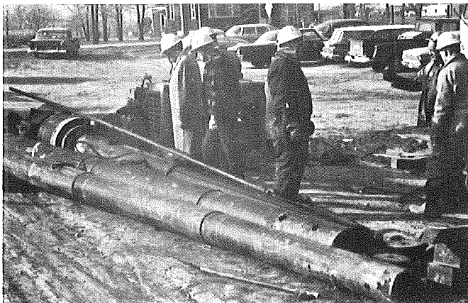
Figure 18. Differential-acting, steam-activated Raymond 15-M (internal hammer). Mandrel is shown at lower left prior to assembly, and cushion component at lower right.
