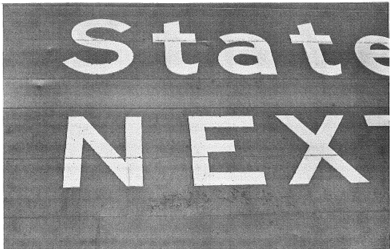
Figure 6. Typical condition of "New" (above) and "Intermediate" (below) signs on I 94.
