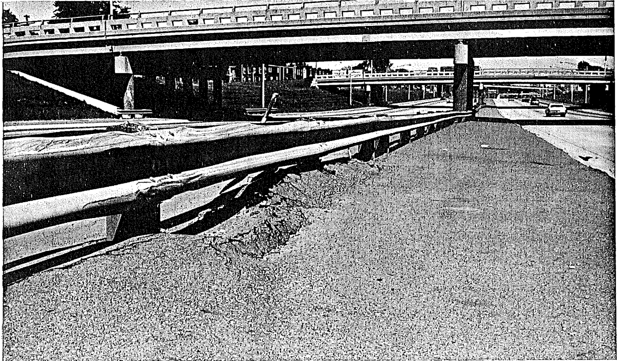
▲ Condition of median in 1969, two years after construction.
