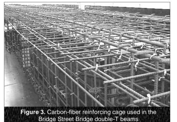
beams to be reinforced with carbon fiber. Straight and bent carbon fiber bars are used for the non-tensioned reinforcement and stainless steel is used for the stirrups. The entire reinforcing cage is assembled similarly to traditional steel cages (Figure 3). The pretension carbon fiber strands are also used in a manner similar to steel pre-tensioning strands in concrete beams. Posttensioning carbon-fiber strands are draped underneath the bridge between the beam webs (Figure 4).
