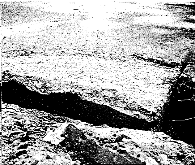
▲ Figure 5. Same break as Figure 3 with joint felt in place and Embeco cement bond coat being applied to lower break.
