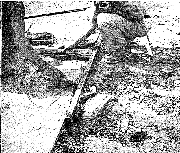
▲ Figure 8. Consolidating grouting mixture in upper corner break.
