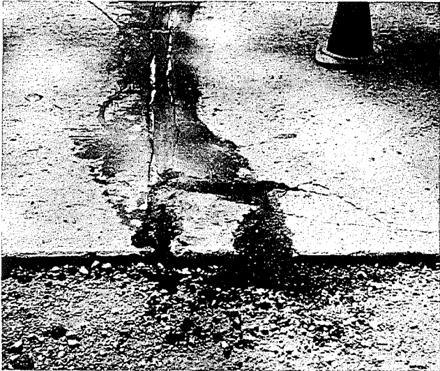
▲ Figure 1. A corner break typical in appearance, having received routine county maintenance treatment.
