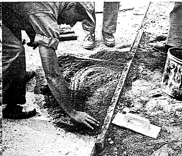
▲ Figure 11. Final finishing of patch. Final picture of series.
