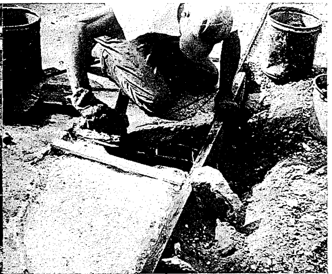
▲ Figure 6. Adding Embeco treated concrete grouting mixture.
