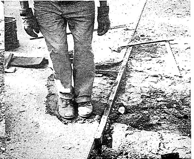
▲ Figure 9. Ready for finish coat.
