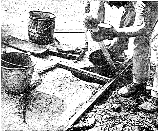
▲ Figure 7. Applying bond coat to upper corner break.
