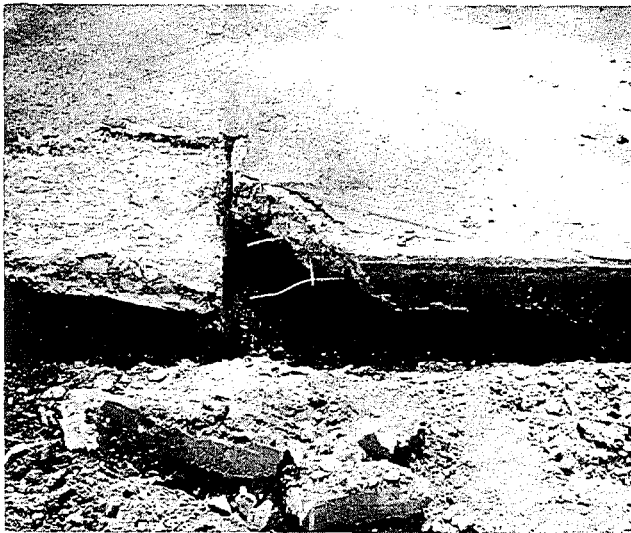
▲ Figure 4. Close-up of top break in Figure 2 with loose and decomposed material removed.
