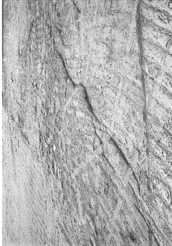
Figure 8. Flowing of Elastizell on sloping fill surface.
