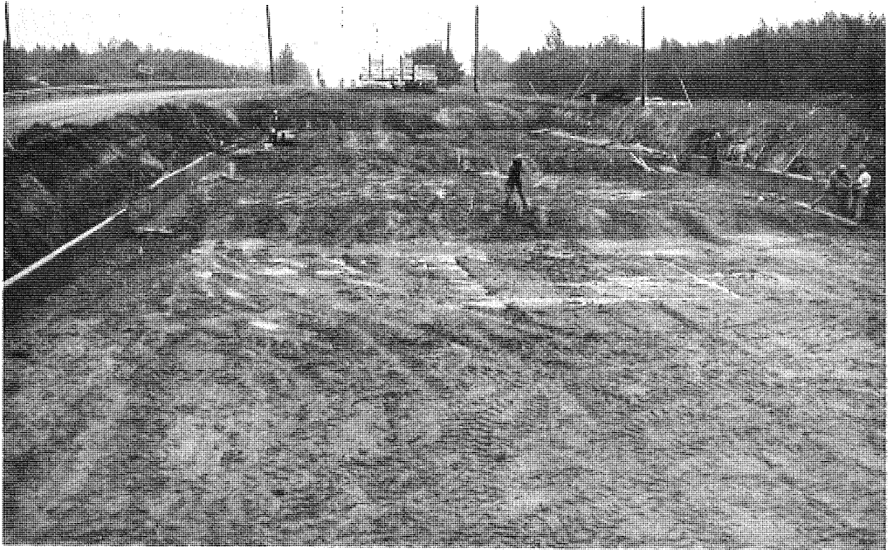
Figure 3. Shaped subgrade prior to pouring Elastizell concrete.
