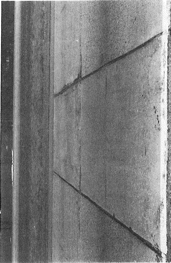
Figure 9. Typical condition of undoweled repairs located within the test section limits.
