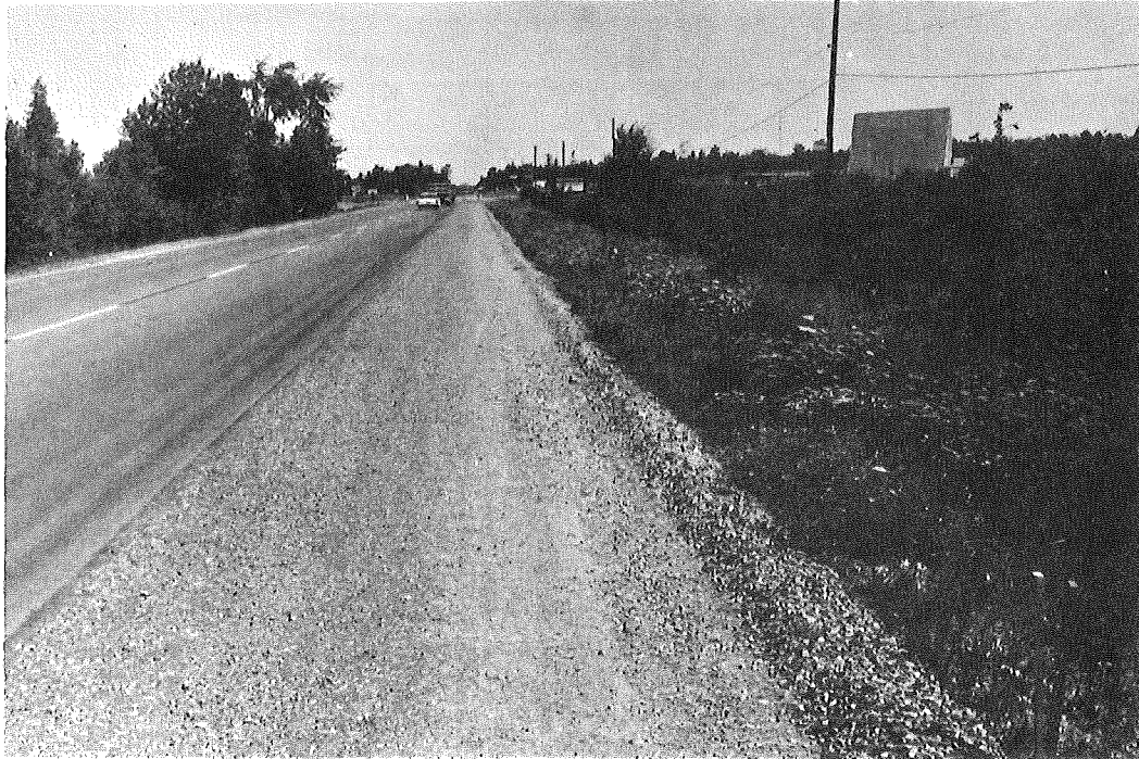
Figure 15. Typical sealed shoulder at completion of operations.
