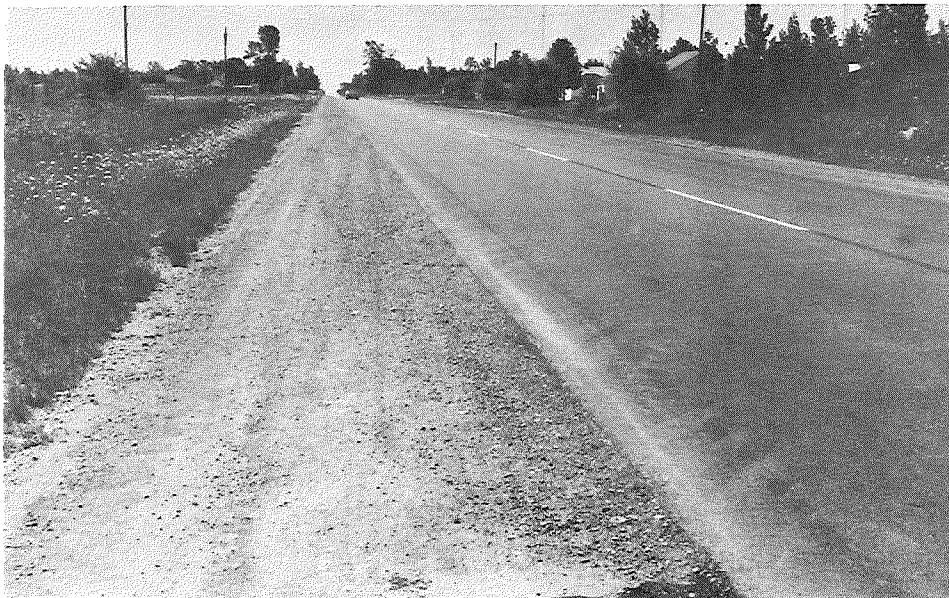
Figure 13. Appearance of the 2-percent asphalt emulsion section.
