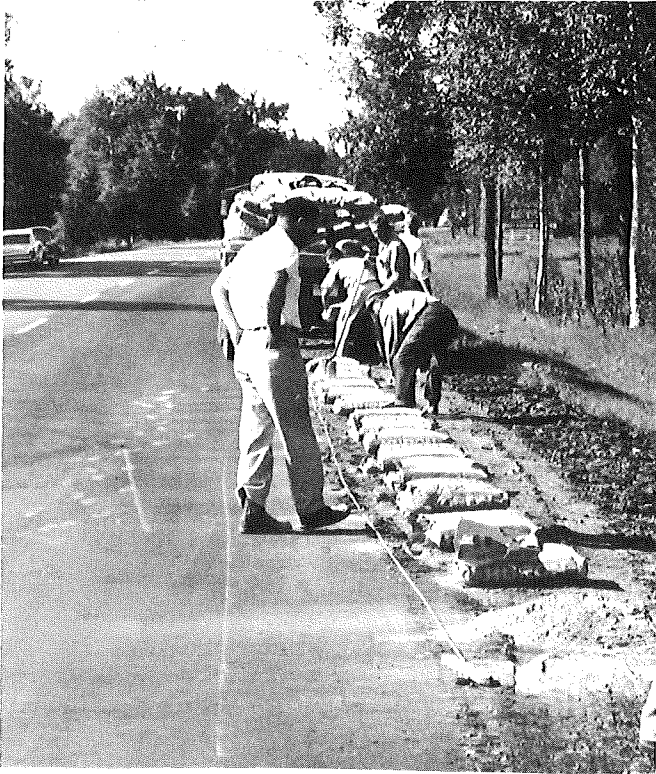
Figure 4. Placing bagged portland cement.
