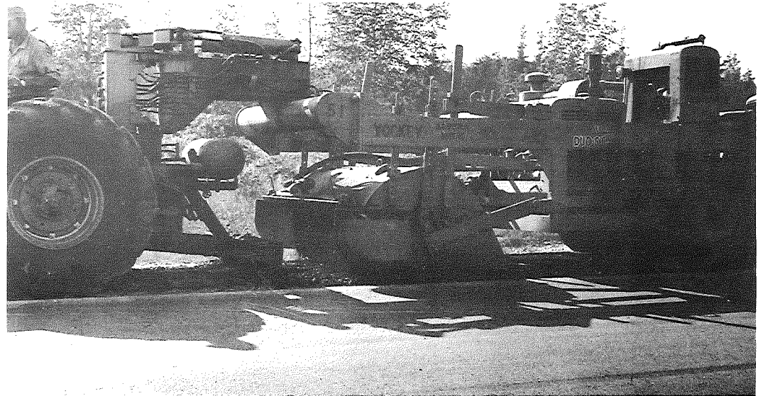
Figure 8. (top left) Moistened shoulder aggregate before application of asphalt for stabilization.
