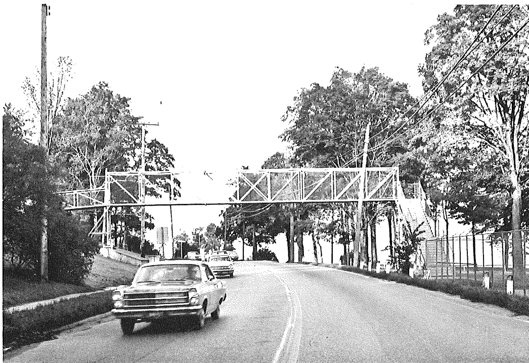
Figure 7. P01 of 24011 over US 31 in East Petoskey. Truss is painted.
