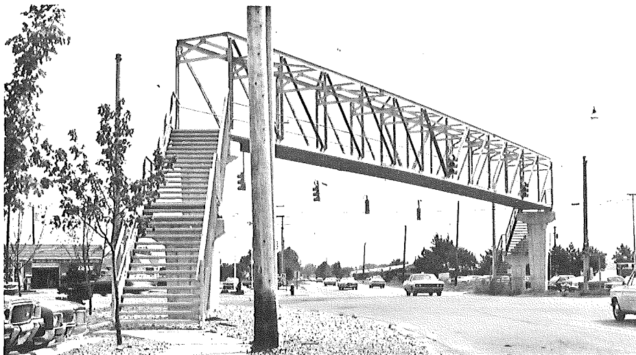
Figure 2. P02 of 50031 over M 97 in Fraser is the test secondary standard (west stairs in foreground). Truss is about 132 ft long.
