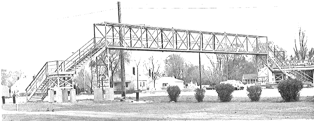
Figure 3. P01 of 50031 over M 97 at Rose Ave in Mt. Clemens. Bridge is galvanized.
