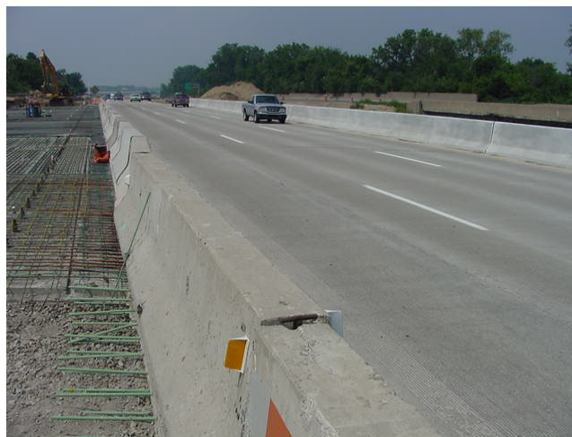
Figure 7 Completed Stage I, R01 of 82022, August 2003.
