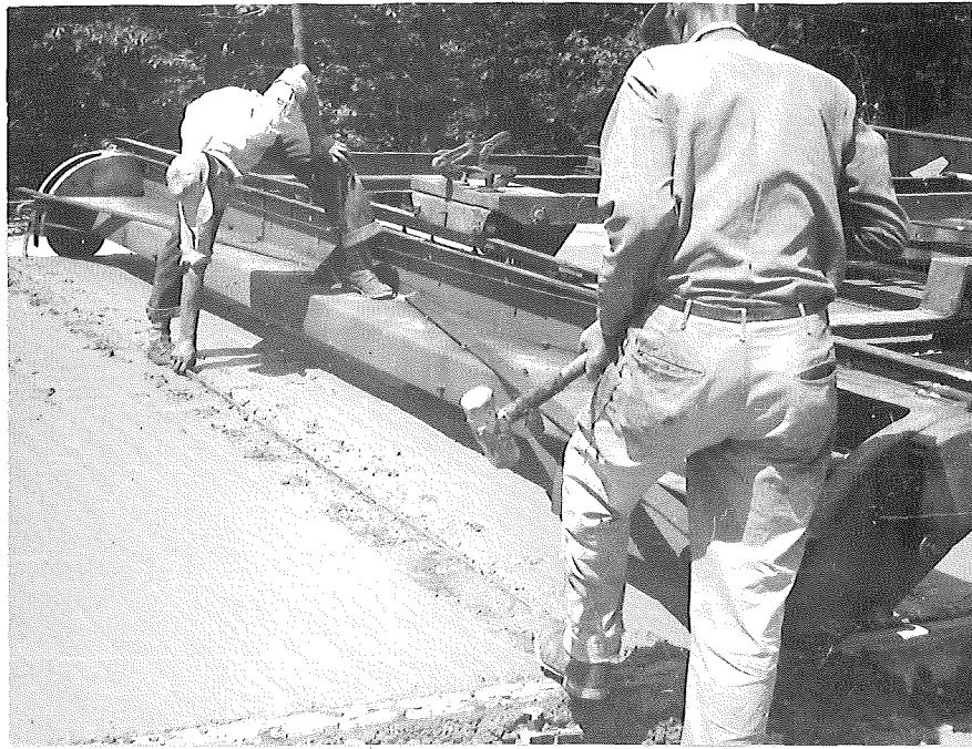
Figure 5. Method of placing steel template to mold contraction joint groove.
