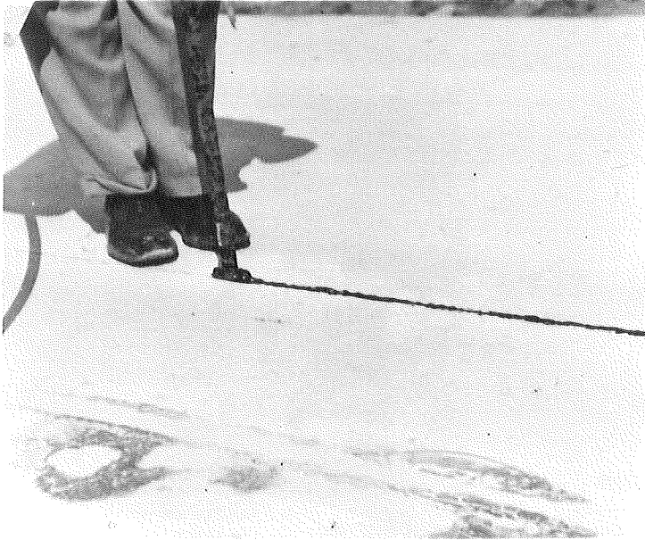
FIGURE 7. APPLICATION OF PRESSTITE NO. 77 TO CENTER JOINT.
