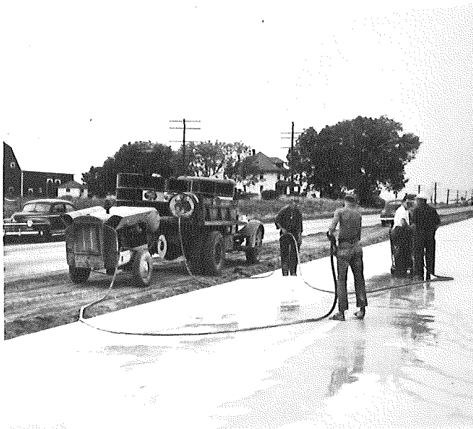
FIGURE 3. OPERATION OF CUTTING LONGITUDINAL CENTER JOINT. NOTE WATER & AIR SUPPLY LINES.
