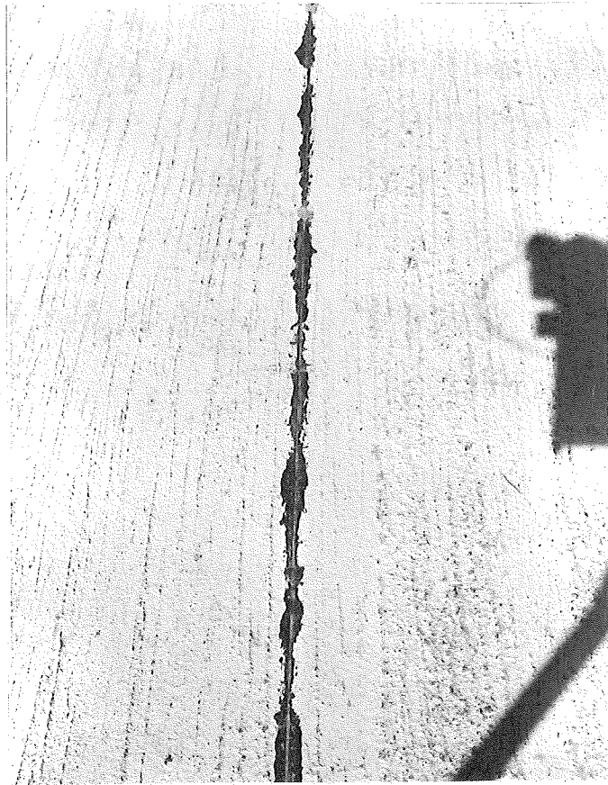
Figure 10. Condition typical of sawed center joint after five months.
