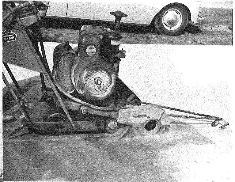
FIGURE 2. CLIPPER SAW, MODEL C-130, USED FOR CUTTING LONGITUDINAL CENTER JOINT.
