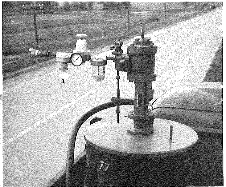
FIGURE 6. PUMPING EQUIPMENT FOR APPLICATION OF PRESSTITE NO. 77.
