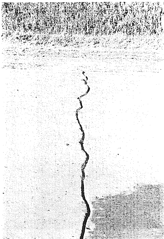
Figure 15. Sawed groove ready for sealant installation.
