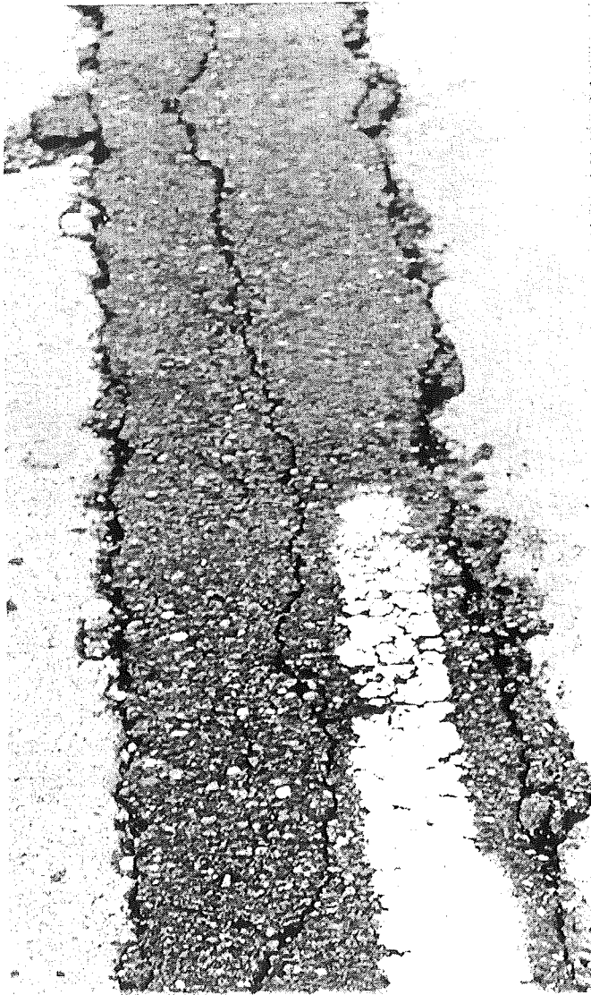
◀ Figure 23. Ravelling along edges and cracking over plane-of-weakness crack--4 years of service.
