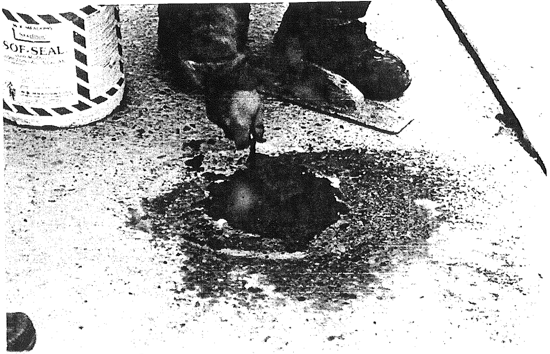
Figure 17. Placing fast-set mortar in pop-out.
