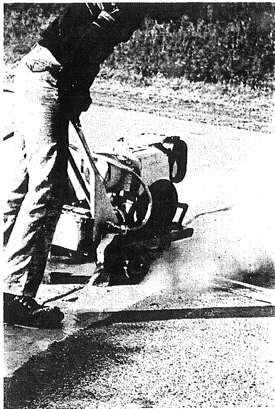
Figure 14. Sawing groove over transverse crack.
