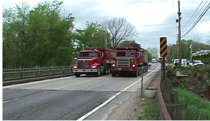
Extreme loading of bridges by heavy trucks in Michigan is much less common than loading by lighter vehicles, which allows for Michigan DOT's modifications to default LRFD/LRFR values.
