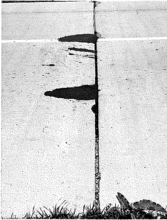
▲ FIGURE 1. SHOWING DISINTEGRATION AS OF AUGUST 3, 1953. STATION 113+21. LOOKING WEST TO EAST.
