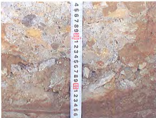
Figure 3. Depth to bottom of existing concrete (at roughly the 35 centimeter mark).
