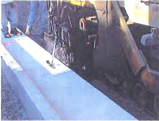
Figure 6. Grade control used for lanes next to curb and gutter.
