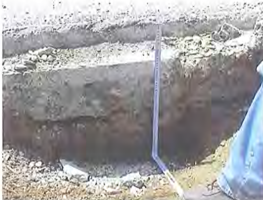
Figure 1. Cross-section of the existing roadway. Red marks on the ruler are every 10 centimeters.
