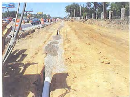
Figure 4. Underdrain in place and partially backfilled.
