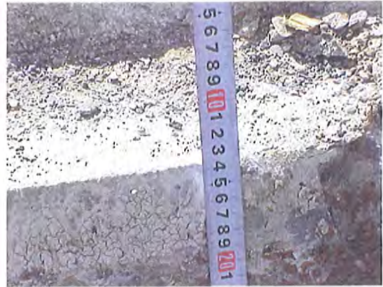
Figure 2. Depth to top of existing concrete.
