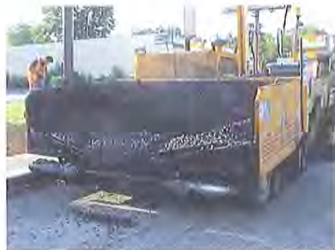
Figure 5. Type of paver used to place the asphalt.
