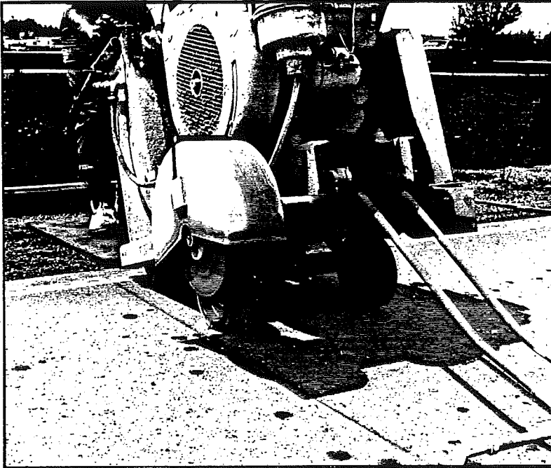
Figure 2. Initial saw cut using dual blades to make parallel grooves 3-3/4 in. apart.
