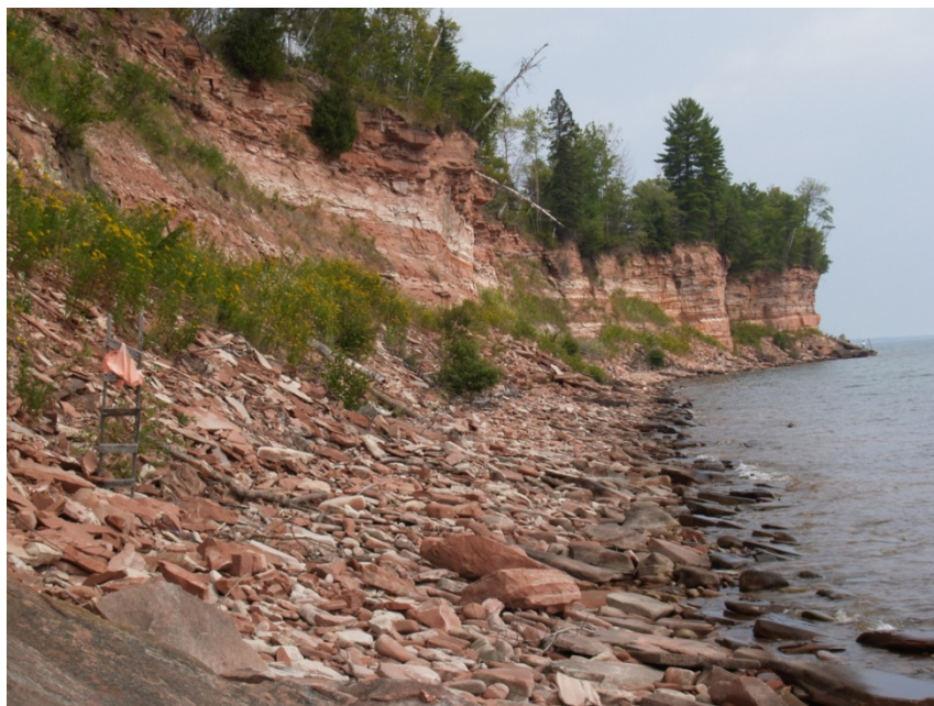
Figure 30 Talus slope just below the section of cliff threatening the highway.
