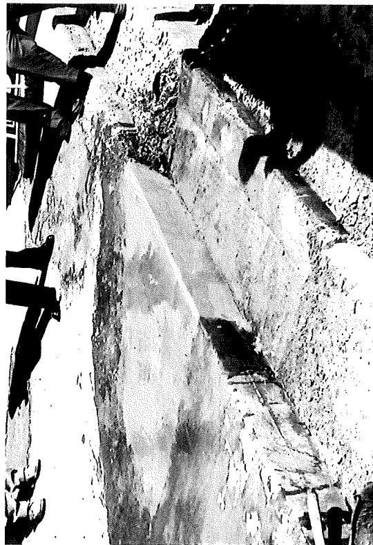
Figure 1. Chipped and pre-wet area before Speed Crete placement (top), and after shaving off excess material and rubbing with wet sponge (bottom). Sidewalk patch on N. Washington Ave., Lansing (4-29-66).
