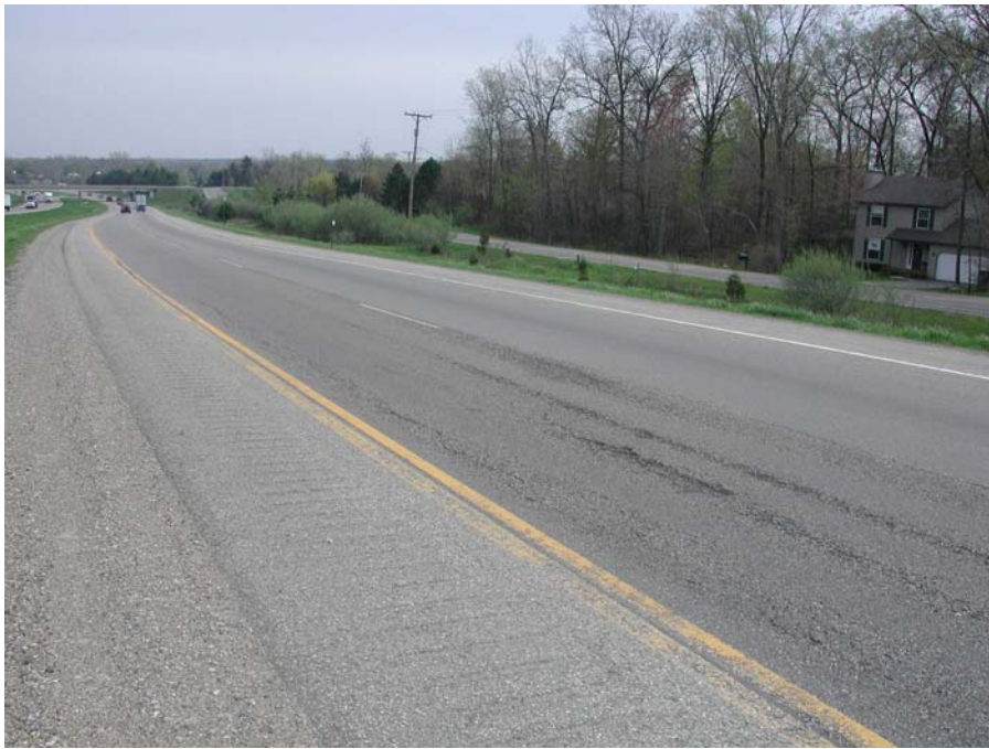
Figure 4.24 Longitudinal TDC and raveling in segregated areas of TDC propagation with depth
