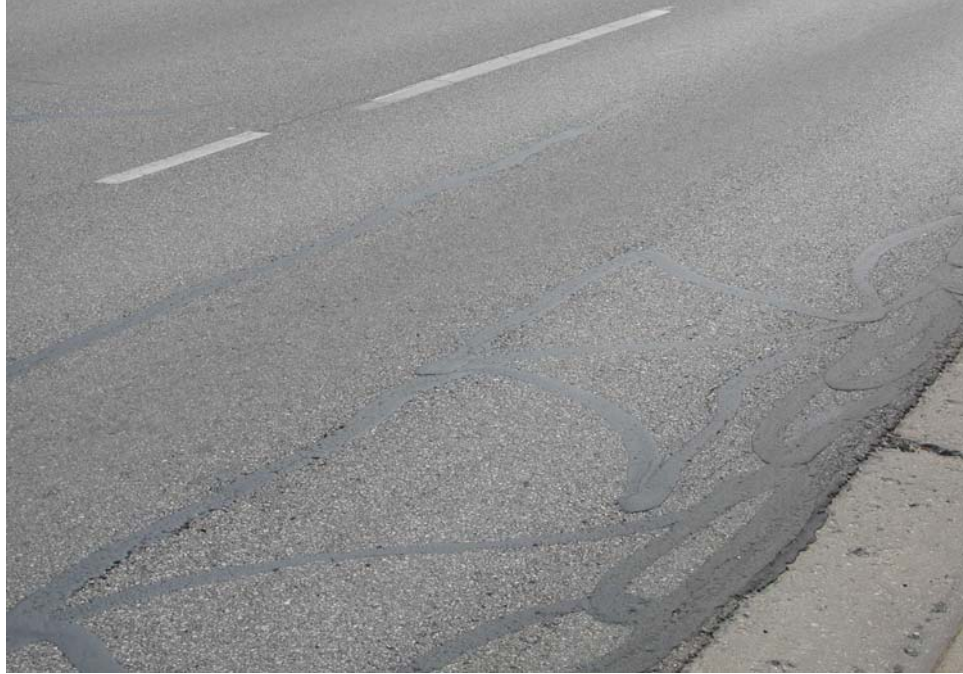
Figure 4.12 TDC in segregated areas at the edge of the wheel path on M-55 (flexible pavement)
