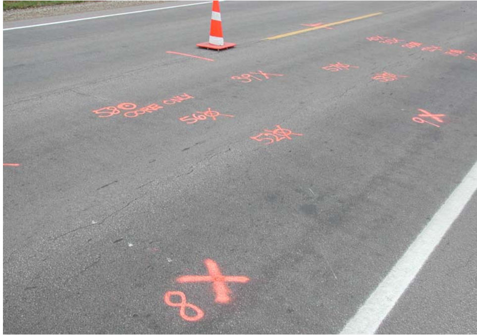
Figure 4.10 TDC on M-50 test section 1 (flexible pavement, no segregation visible)
