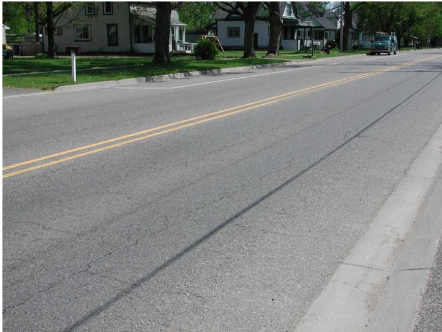
Figure 4.20 The third stage of TDC development, LTDC and TTDC forming a networks on East Michigan Avenue, control section 39555 job number 39212, May 2002
