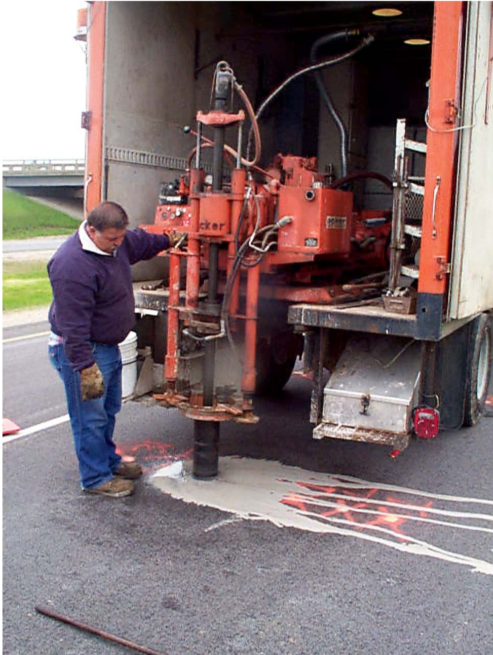
Figure 3.5 Drilling cores using a power rotary drill
