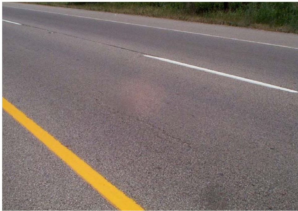
Figure 4.5 TDC initiation at the edge of the wheel path on M-20 (flexible pavement, no segregation is visible)
