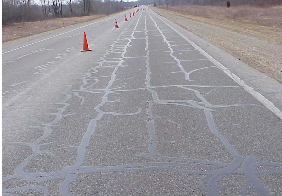
Figure 4.6 Advanced level of TDC on M-37 (rubblized pavement)
