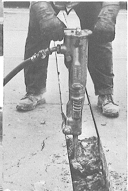
Figure 4. Removing concrete between narrowly spaced saw cuts with air hammer.
