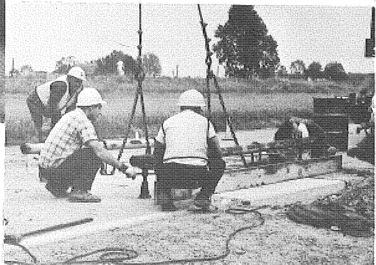
Figure 17. Establishing final elevation of pre-cast slab by adjusting jacks. The jacks were left in place until mortar had set sufficiently to carry the slab.
