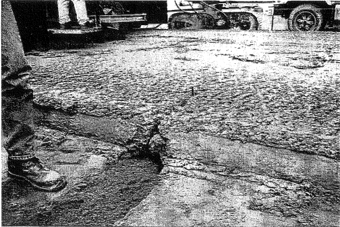
Photo C39. A view of the thermocouple rig immediately after installation in CSN# 47065-28215A WB. The rig is installed between paving lifts, and the cables are buried to protect them from damage during the second paver pass.
