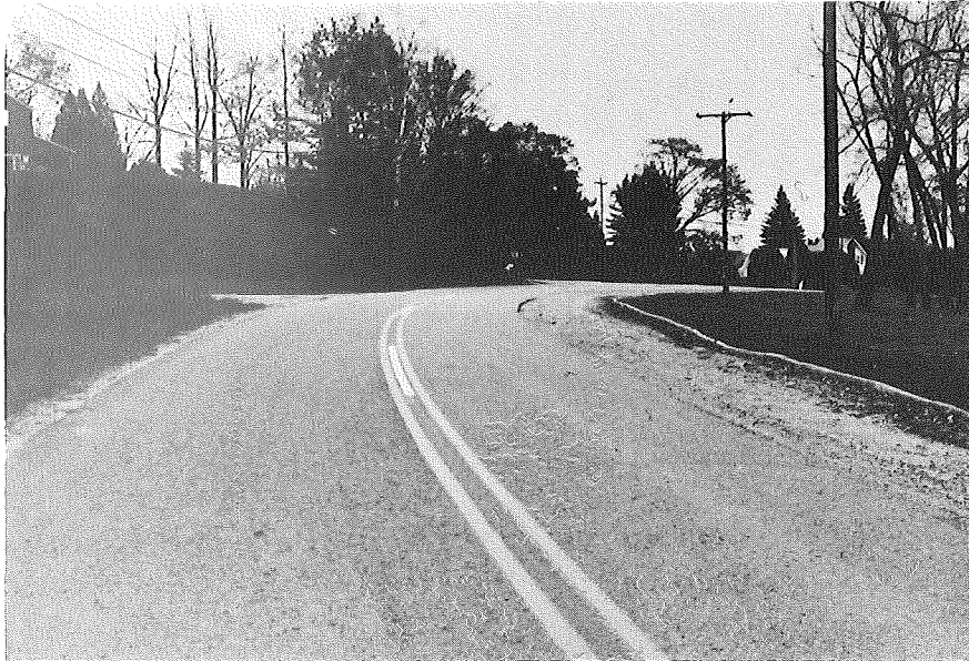
SOUTHBOUND CRYSTAL ROAD APPROACHING THE INTERSECTION
