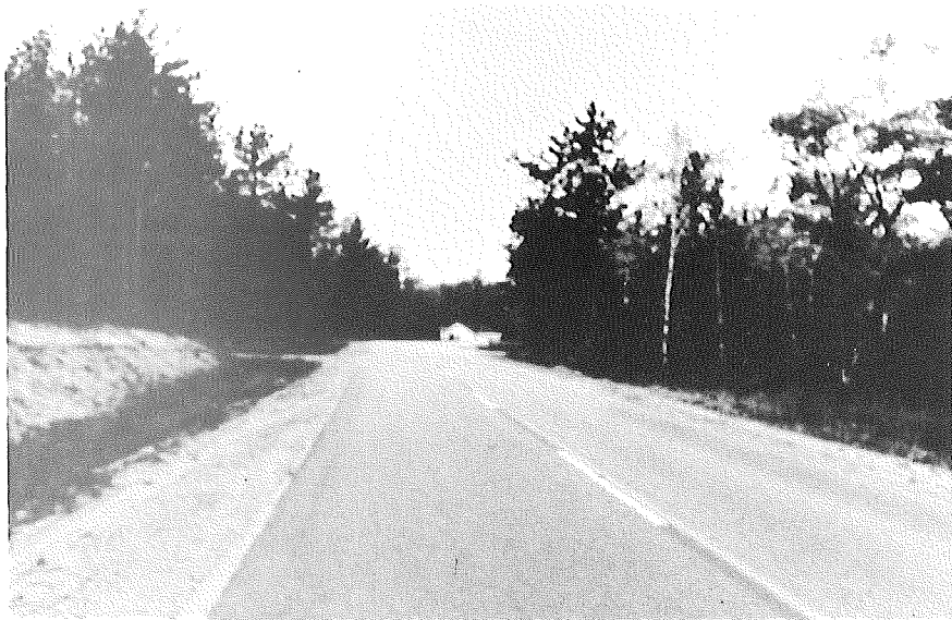
WESTBOUND LAKE MICHIGAN ROAD
