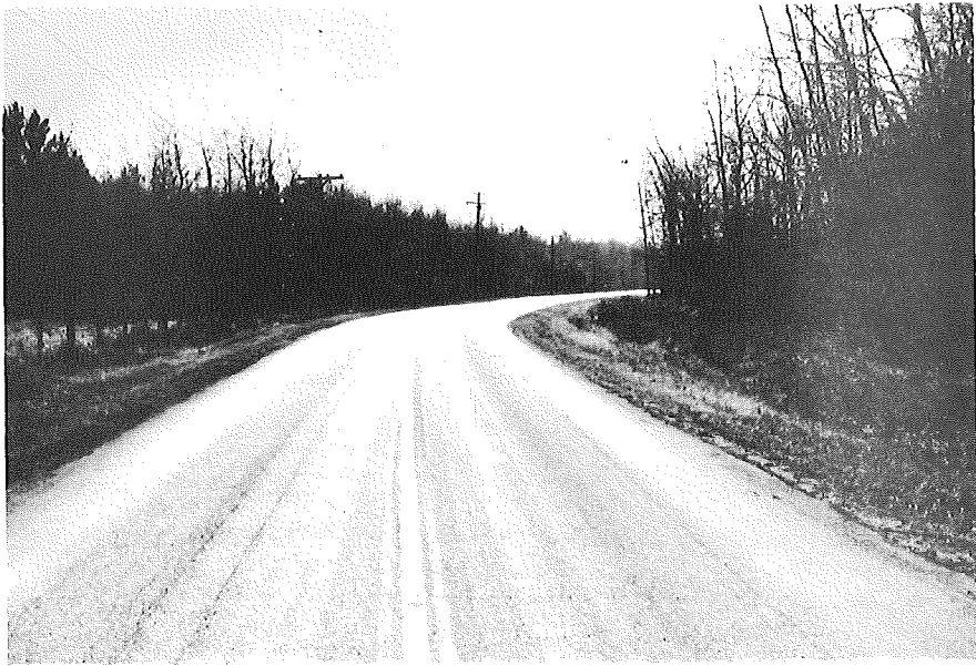
SOUTHBOUND INDIAN HILL ROAD APPROACHING THE CURVE
