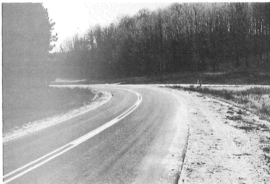
WESTBOUND NARROW GAUGE ROAD AT THE INTERSECTION
