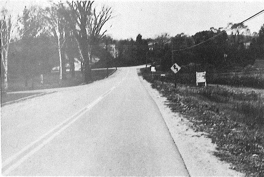
NORTHBOUND CRYSTAL ROAD APPROACHING THE INTERSECTION
