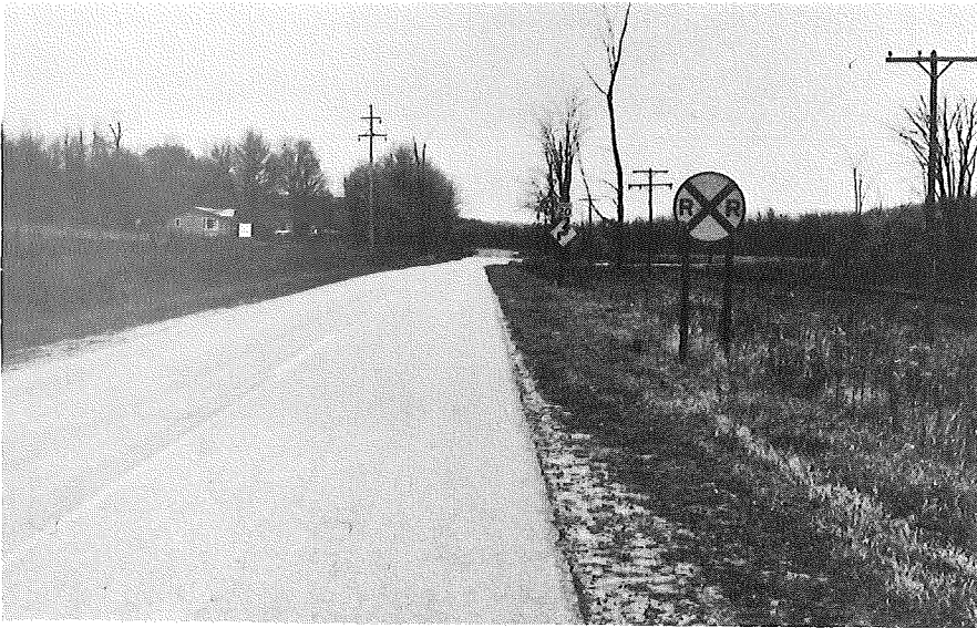
EASTBOUND RIVER ROAD APPROACHING THE INTERSECTION
