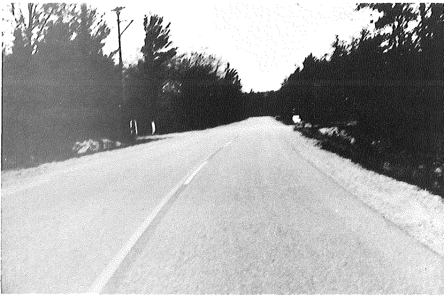
WESTBOUND LAKE MICHIGAN ROAD
