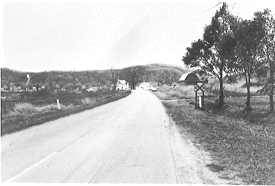
WESTBOUND RIVER ROAD APPROACHING RAILROAD CROSSING
