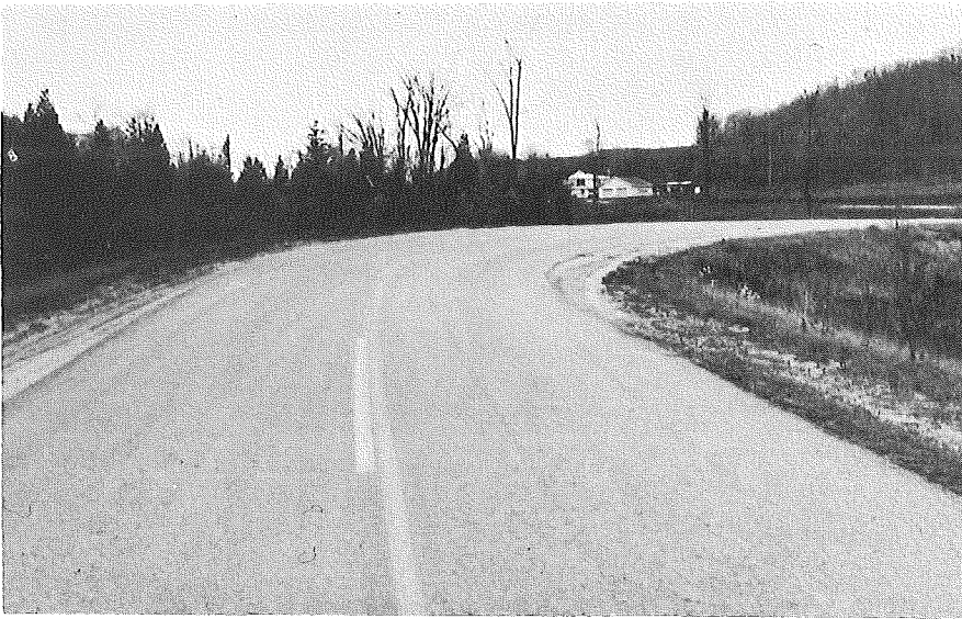
WESTBOUND RIVER ROAD APPROACHING THE INTERSECTION
