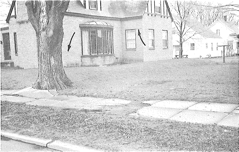
General view showing some major fractures
