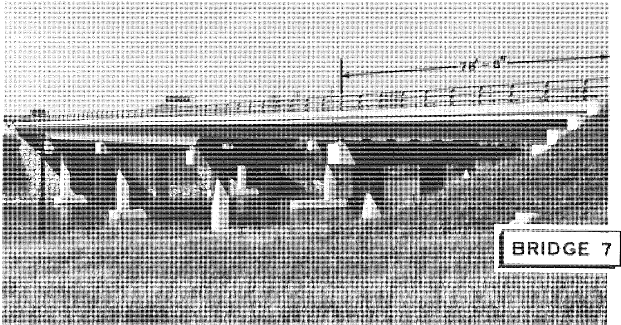
Bridge 7: Simple span, rolled beam with tapered end cover plate
