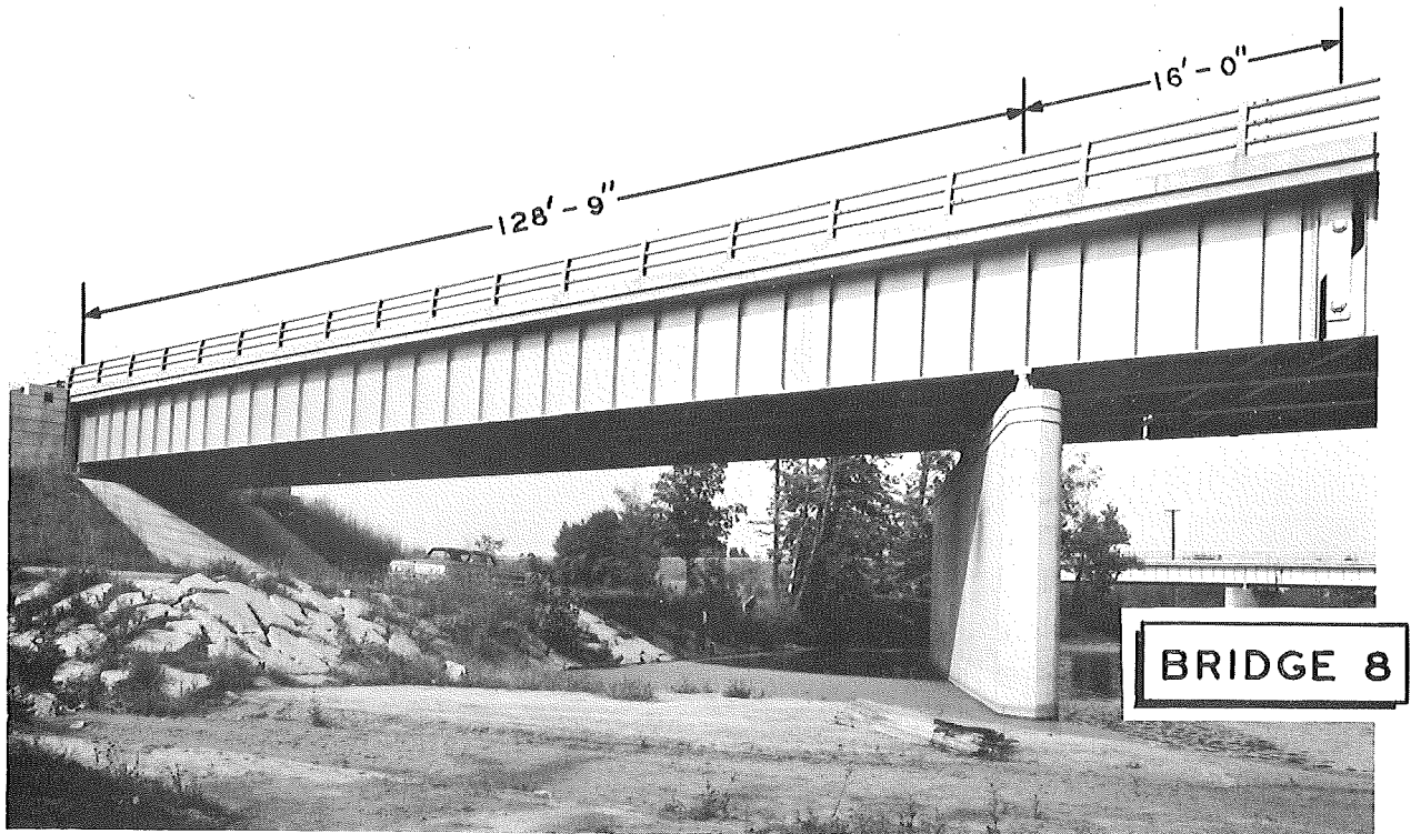
Bridge 8: End anchor span, welded plate girder with flange thickness transition
