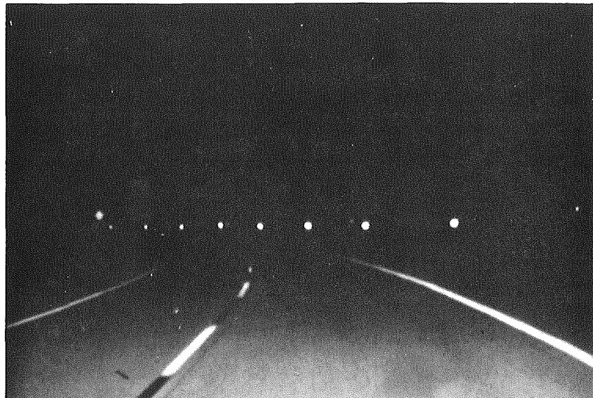
SITE #1 AFTER EDGELINING - Left curve
