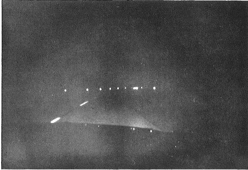
SITE #2 BEFORE EDGELINING - Right curve
