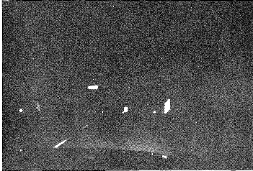
SITE #3 BEFORE EDGELINING View ahead under M-36
