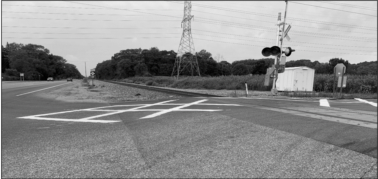
Figure 5. Dynamic Envelop Crosshatching at M96 and 28th Street (Source: MDOT).
