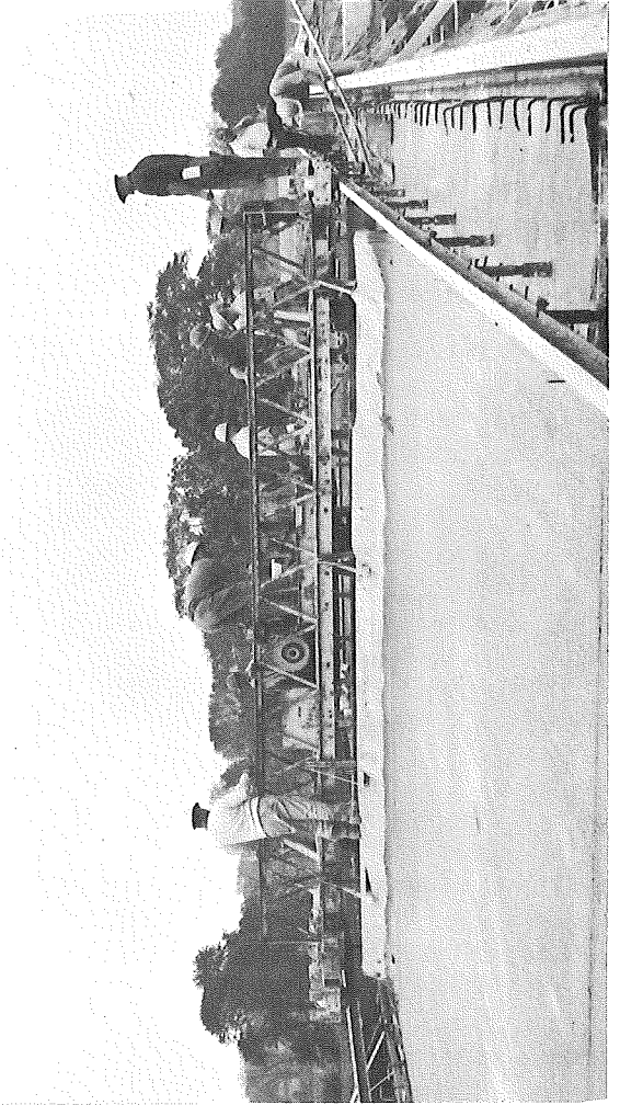
Figure 2. View of elevating, placing, and finishing concrete at the Coe Rd. site.
