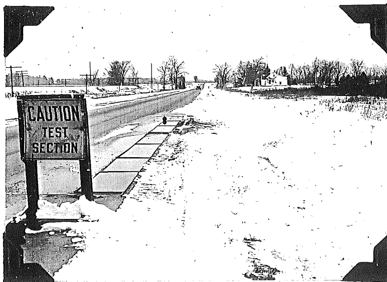
Figure 1. Typical installation of test panels.
