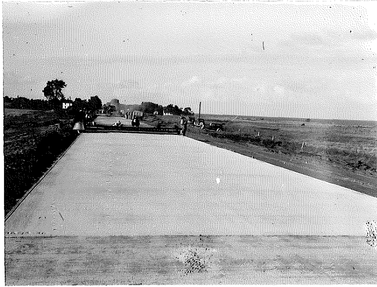
Figure 1. General view of curing project looking north from Station 1067+52.
