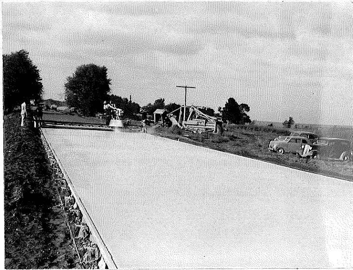
Figure 11. Another view showing uniformity of application with double pass and new nozzles.
