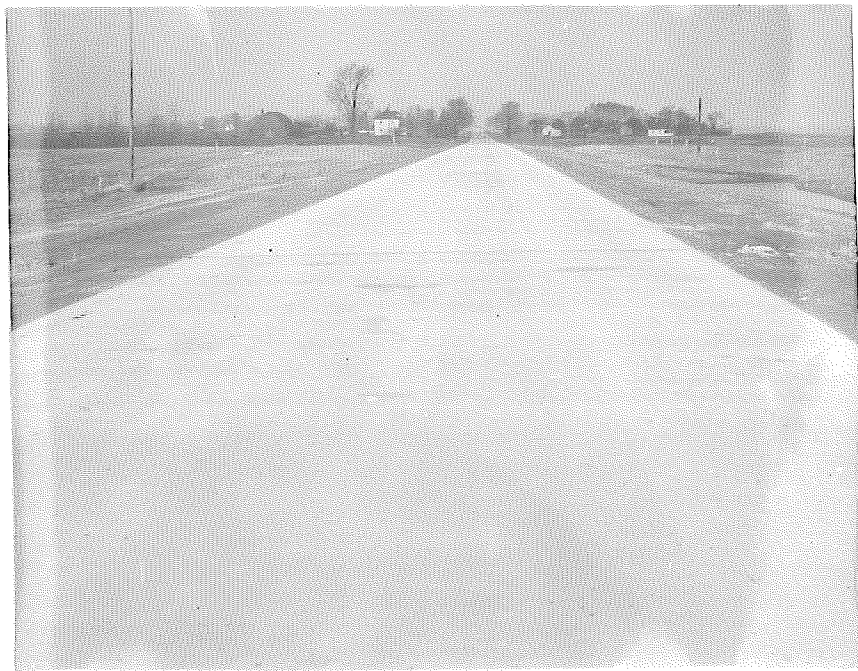
Figure 12. Looking north from beginning of project; 8 weeks after application. Intermediate color in center of picture is due to spraying white membrane on day-old concrete.
