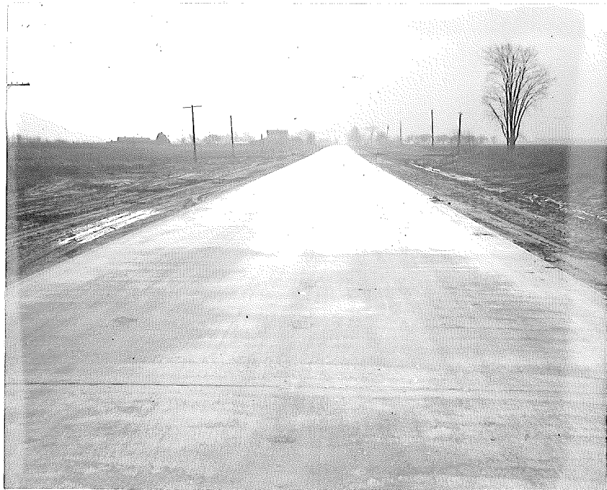
Figure 14. Looking south into the end of curing project. Sun in front of camera. Contrast is more evident when looking into the sun.
