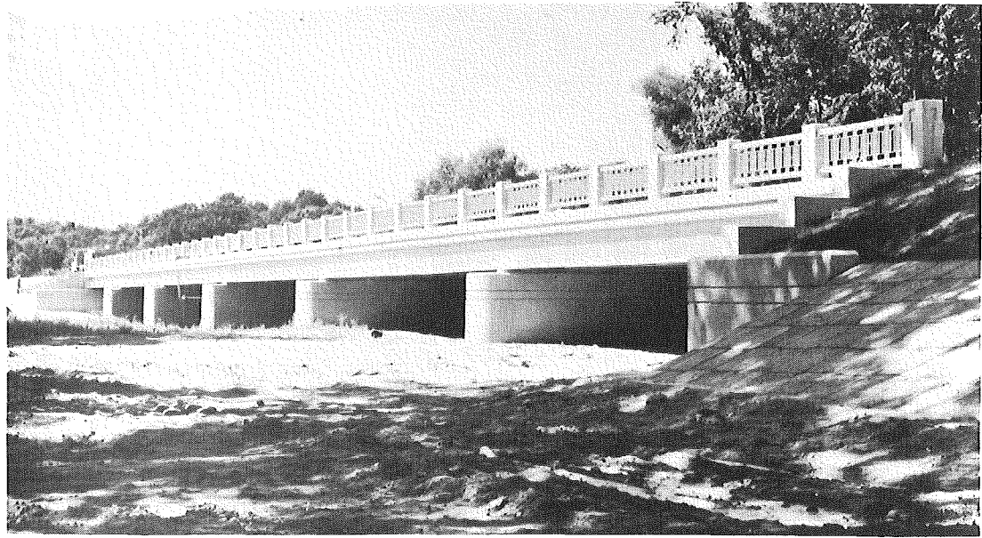
▲ FIGURE 20- GENERAL VIEW OF FENNVILLE BRIDGE.
