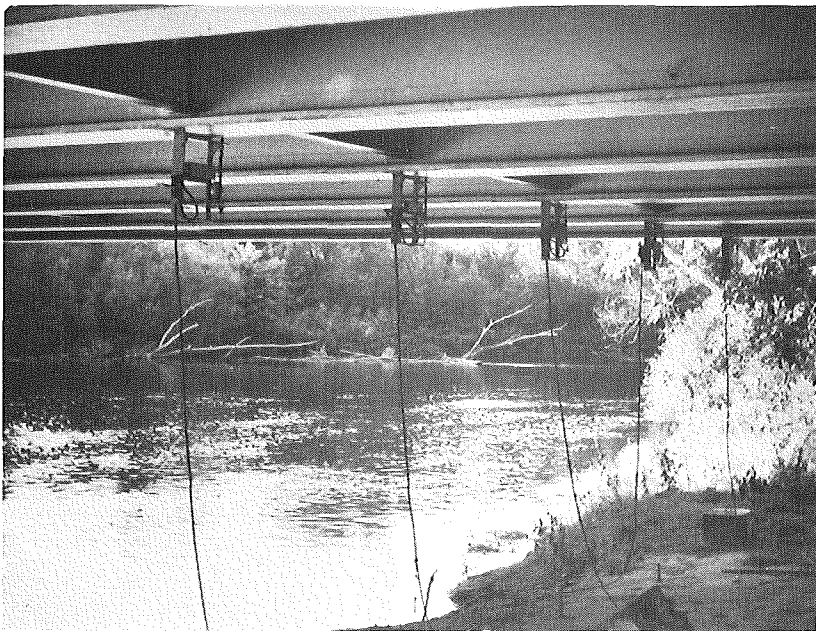
▲ FIGURE 21- DEFLECTOMETER INSTALLATION, SPAN 4.
