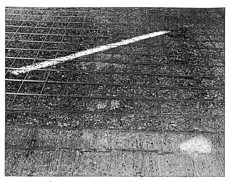
Figure 5. Scaled and abraded area at south end of lift span.
