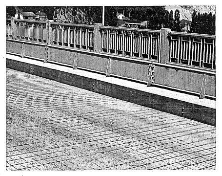
Figure 2. Outside curb showing no welds to roadway bars and variable gap between curb and deck.
