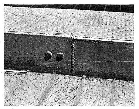
Figure 1. Median curb showing welds on transverse steel and gap along bottom between curb and deck.
