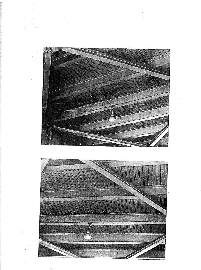
Figures 3 and 4. Two adjacent bays showing deck leakage, dark areas, causing corrosion along top of center stringer (supporting light fixture).
