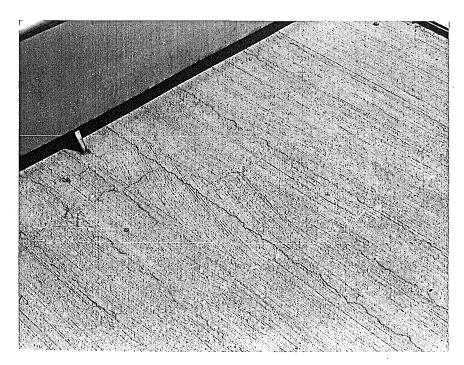
Figure 6. Concrete filled, steel T-grid walk showing typical crack pattern.
