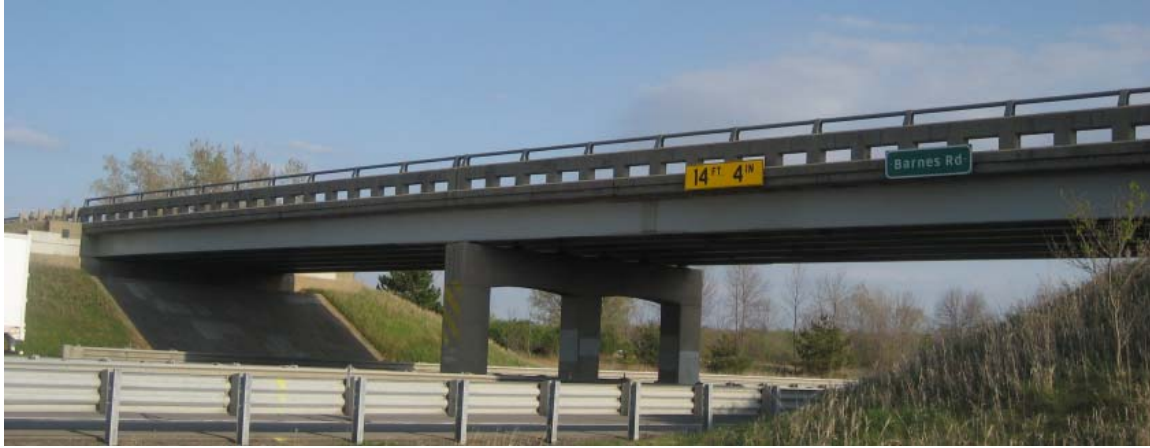
Figure 6.10 Barnes Road over US127 (Bridge 1)
