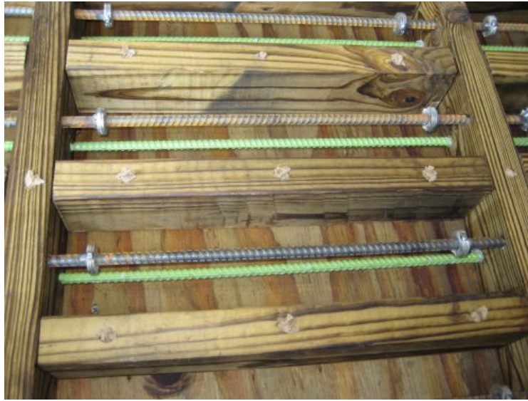
Figure 2.6 Molds before Casting
