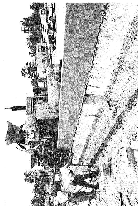
Figure 3. Construction of the glare screen (left) and finished product (right).
