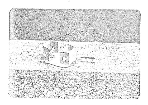
Heavier Bracket and 3/8 inch Anchor Bolt
