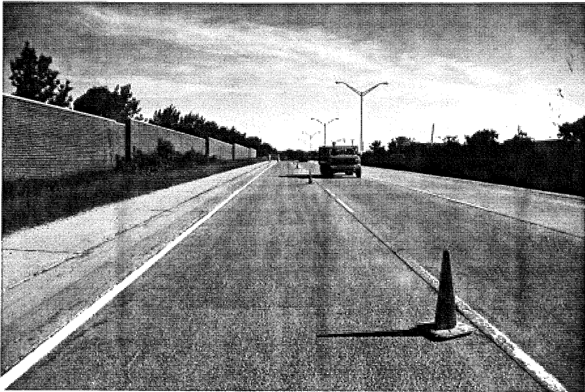
Photo C29. An overview looking north on CSN# 25132-06582A SB. This photo shows the 3 lanes of traffic and the third point intermediate shoulder joints. The slab length is 44 ft in the driving lanes.
