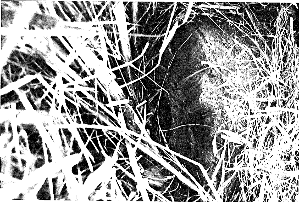
Photo C48. A drainage outlet structure partially clogged with vegetation and debris on CSN# 77024-20821A Section A, EB.
