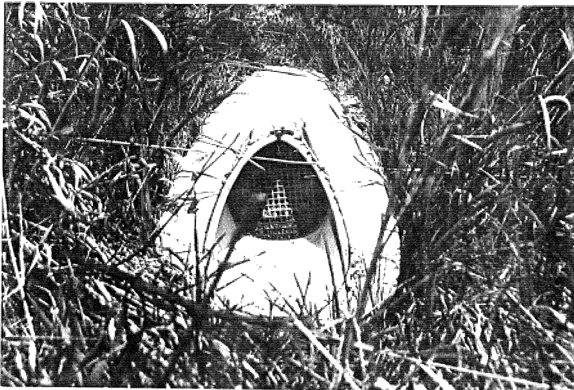
Photo C4. A typical drainage structure of CSN# 11017-32516A (Section A), EB. Water can be seen flowing freely from the drain after coring.
