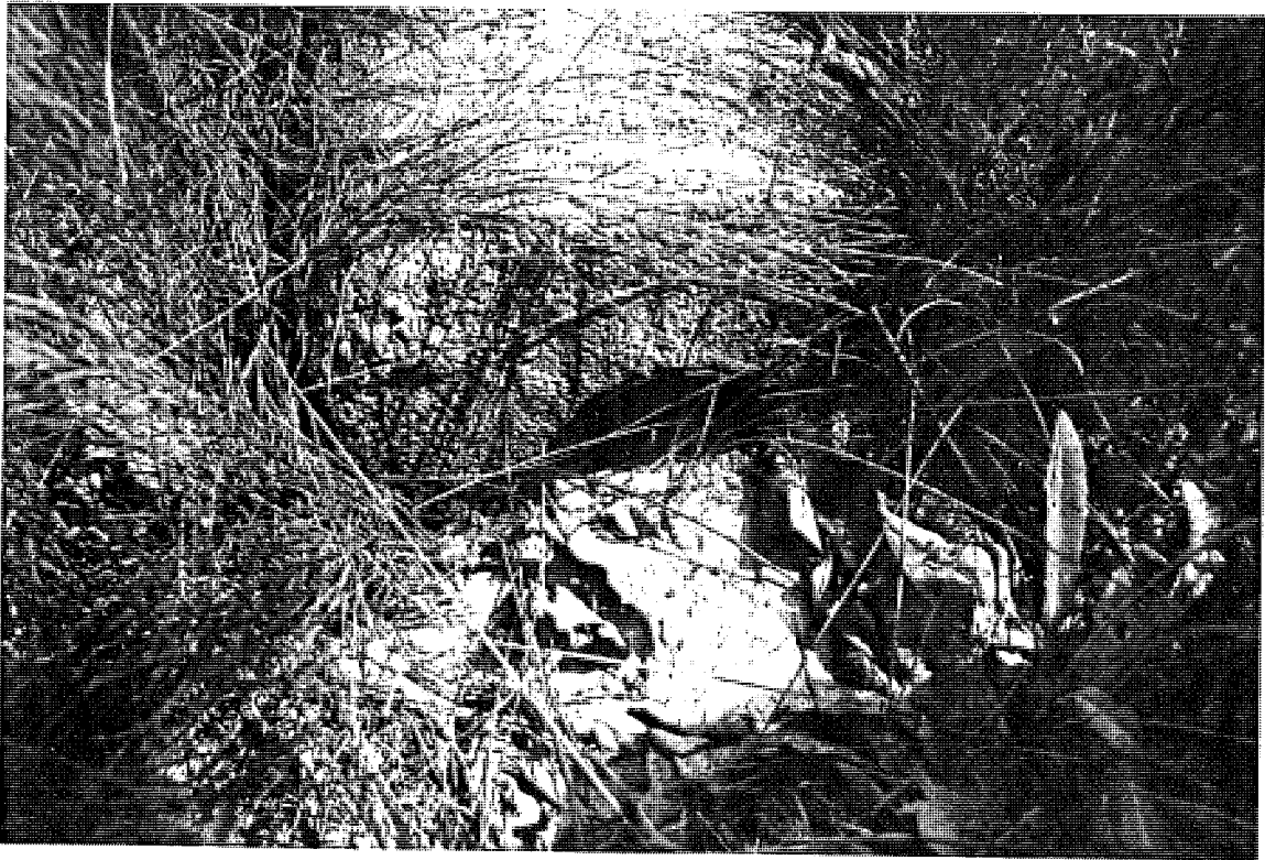
Photo C44. A drainage structure that is clogged with sand and debris on CSN# 77023-21586A EB.
