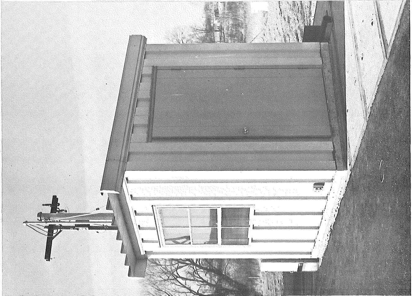
Figure 10. Shoulder enclosure erected to house electronic components removed from pits and truss junction box, and additional Part B equipment.
