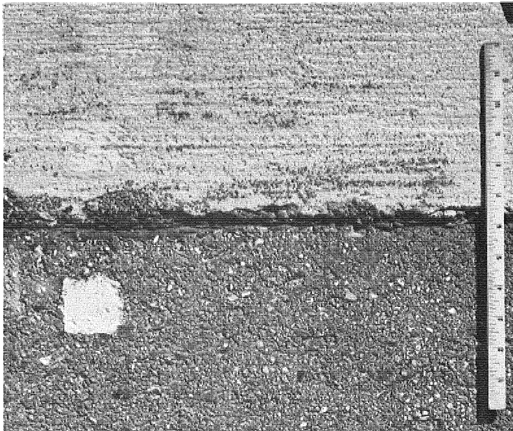
Station 404+60 SB Roadway Age - 1 year 5 months
