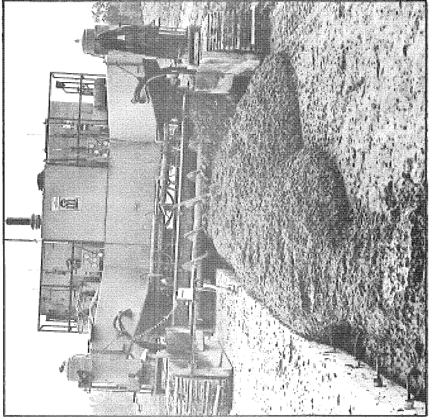
Figure 5. Twelve-ft CMI slip-form paver used to place 9-ft concrete shoulder on I 69 near Charlotte, Michigan.
