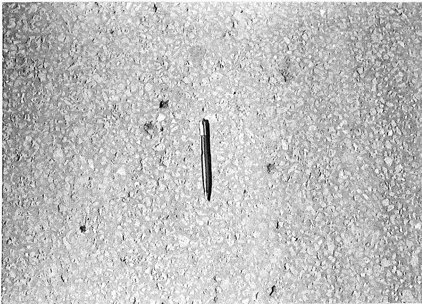
Figure 23. Bituminous concrete resurfacing on Front Street, Traverse City, 400 block. New pavement put down in 1945. Test area 28.
