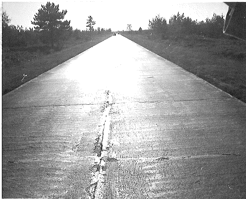
Figure 5. Stone sand concrete. Typical appearance of smooth surfaces under reflected light.
