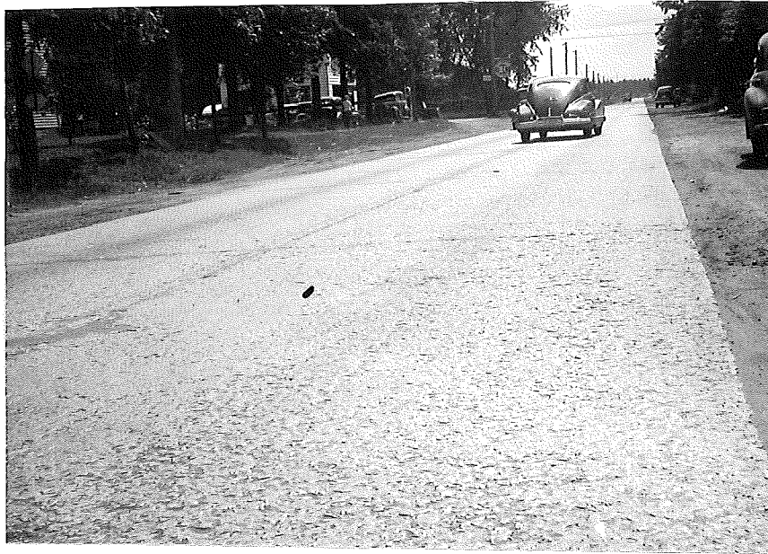
Figure 6. View of Inland stone sand concrete. Completely scaled area. US-2 in Manistique.
