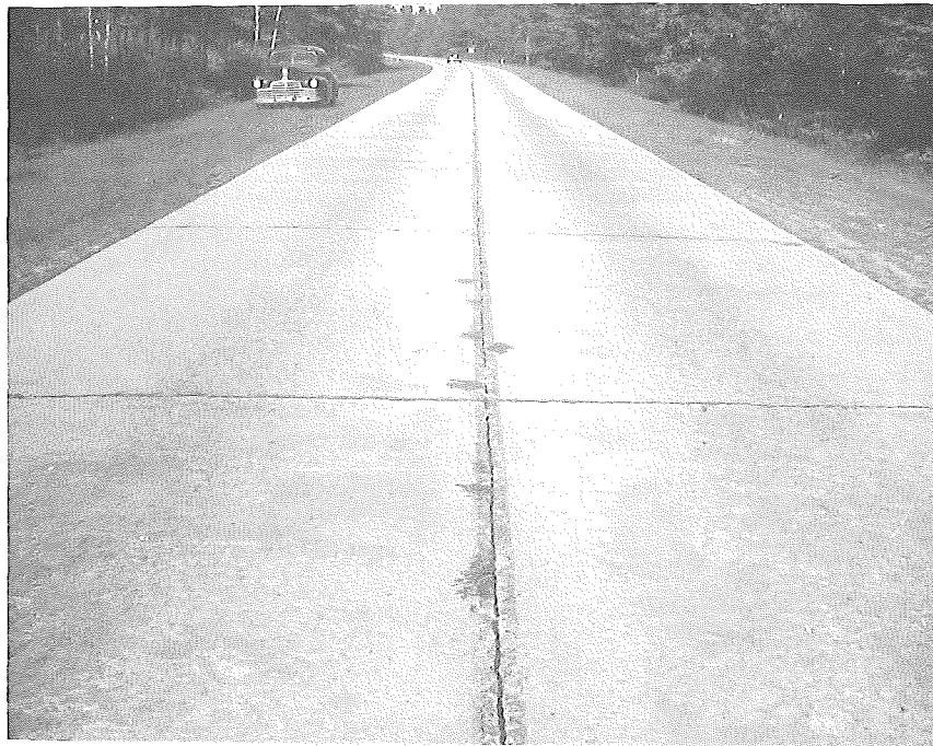
Figure 11. General view of curve at Cooks Corners. F 75-30, C5.
