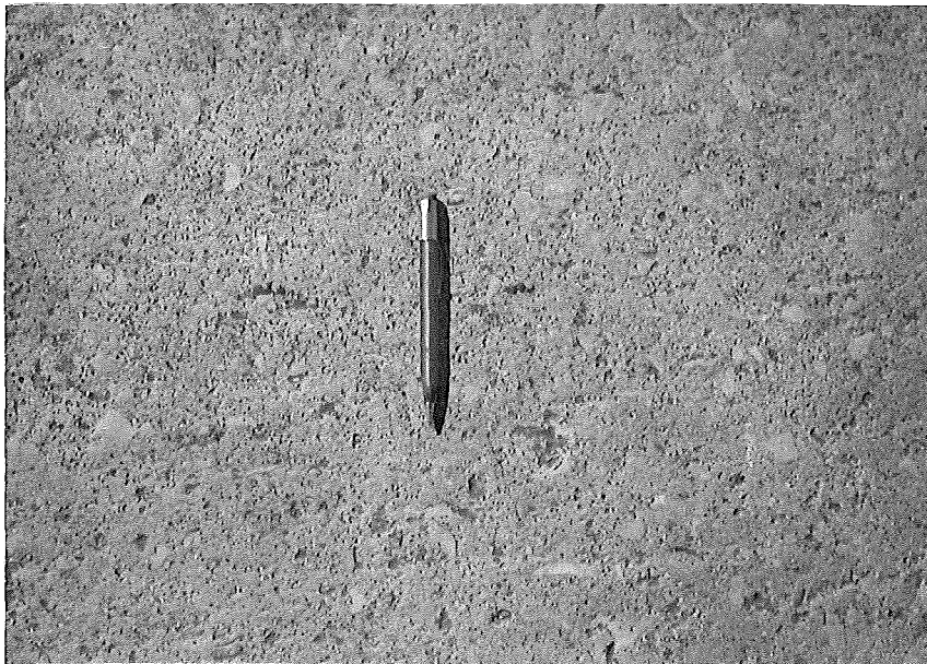
Figure 21. Stone sand concrete on US-31 at M-110, Manistee, Project 51-2, C3-5.
