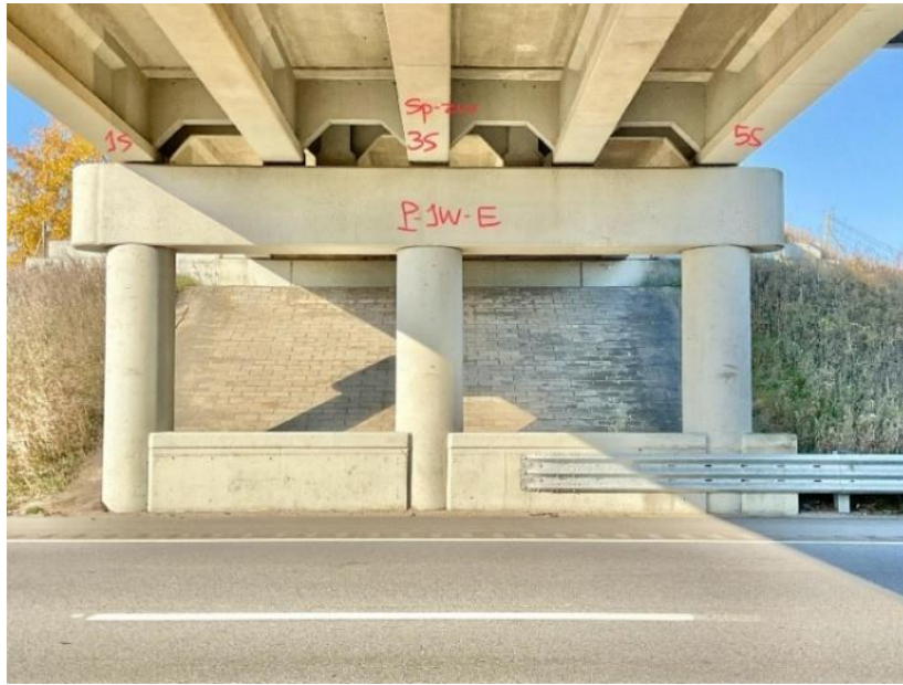
Figure 3-3. Bridge image (H(32).jpg) used for semantic segmentation.
