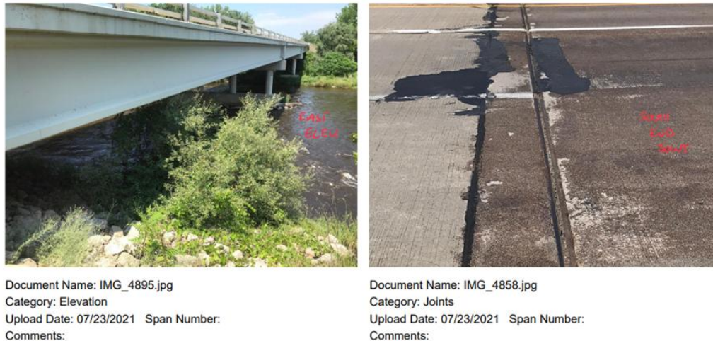
Figure 2-3. Inspection images in MiBRIDGE, the bridge and culvert management system.
