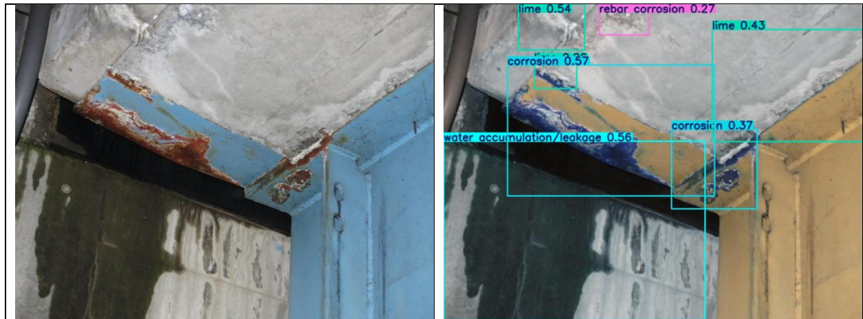
Figure 3-16. Detection of damage in a steel beam bridge.
