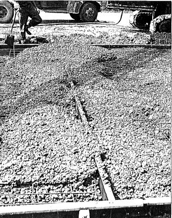
Construction practice adjacent to joints, showing how concrete must pass freely through mesh without segregation to insure satisfactory work.
